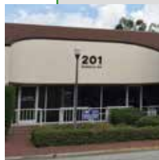
Pictured, above and left: Central Florida Health Care will renovate 4 locations simultaneously with financing through the NMTC Program.
